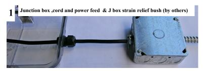
**To make electrical connections**: Pull power cord (by others) through supplied watertight strain relief gland and tighten making sure there is a watertight seal.
